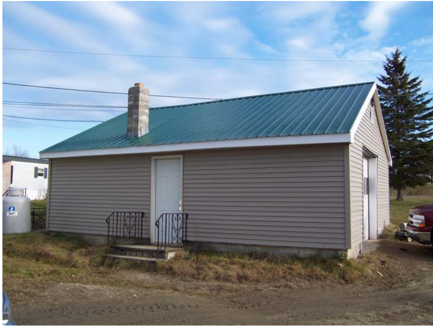
Figure 4-1. Pre-Existing Treatment Building at Spring Brook Mobile Home Park
