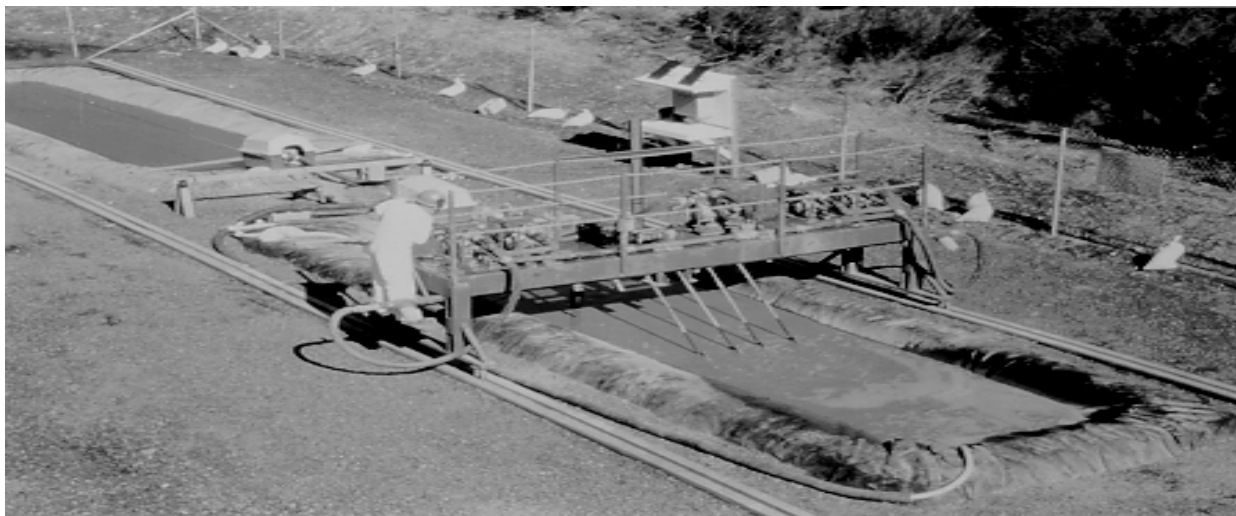
Bioreactors and Soil Mixing System at a TNT-Contaminated Site in Washington
