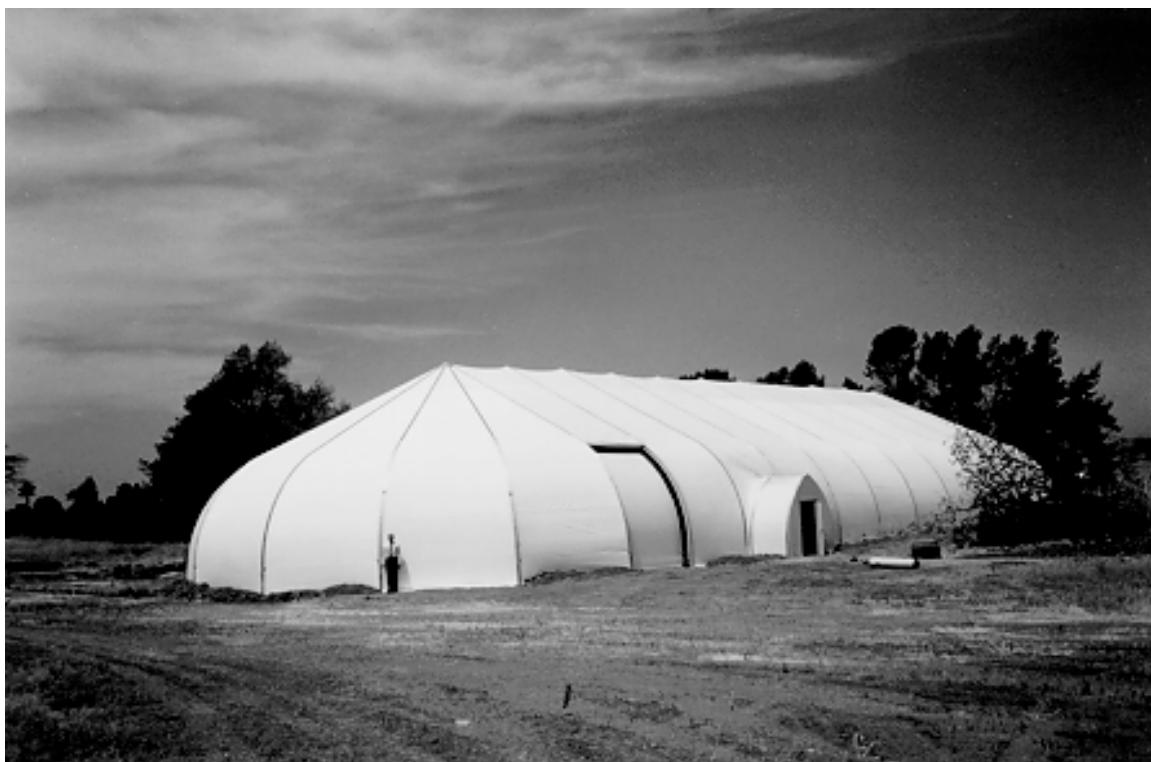
Excavation Area Enclosure
