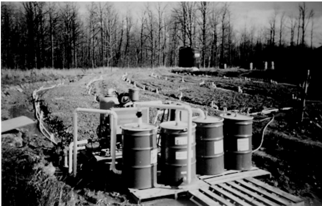
In Situ Bioventing Treatment System
