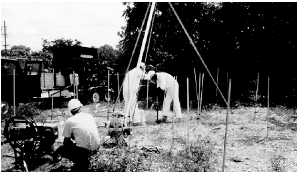
Hydraulic Fracturing Process (Well is at center of photograph)
