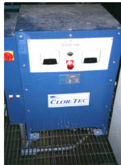
Photograph 2.4 Power Supply/Rectifier
