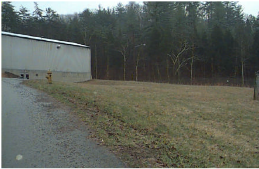
FIGURE 3: Field area where demonstration will be conducted. The structure in the corner of the picture is Building 5507.
