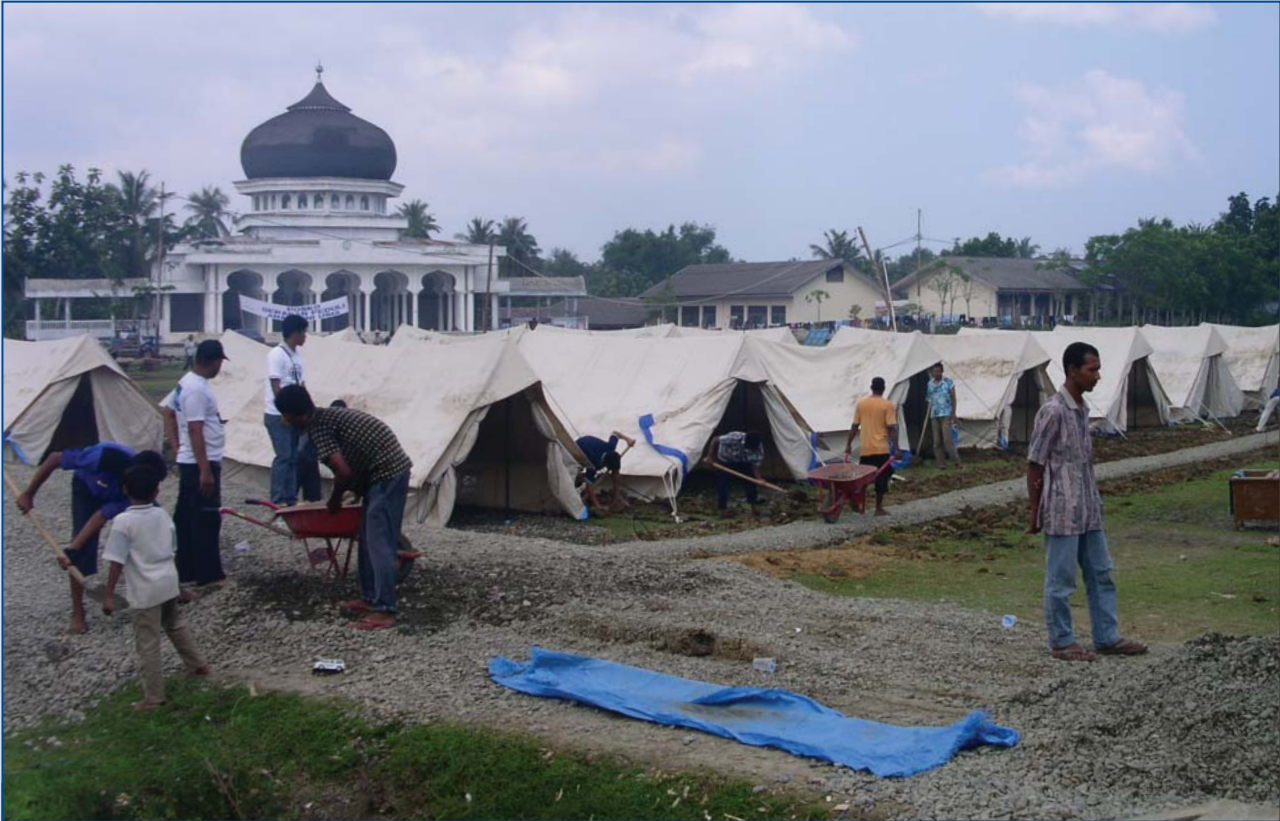
OFDA partner IRD manages water and sanitation activities at a temporary shelter site in Aceh Province, Indonesia.
