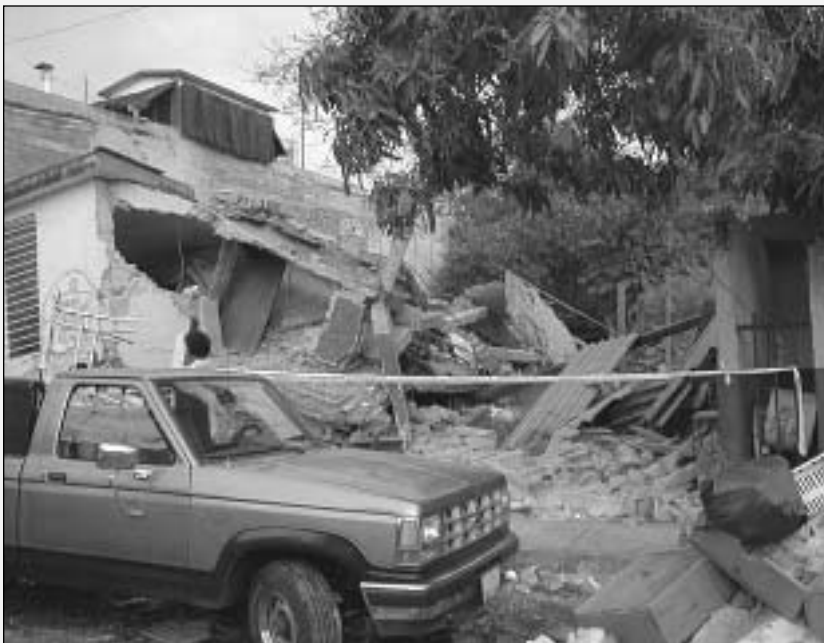
Structure that collapsed following the January 21, 2003 earthquake in Colima, Mexico (photo by Tim Callaghan, USAID/OFDA).
