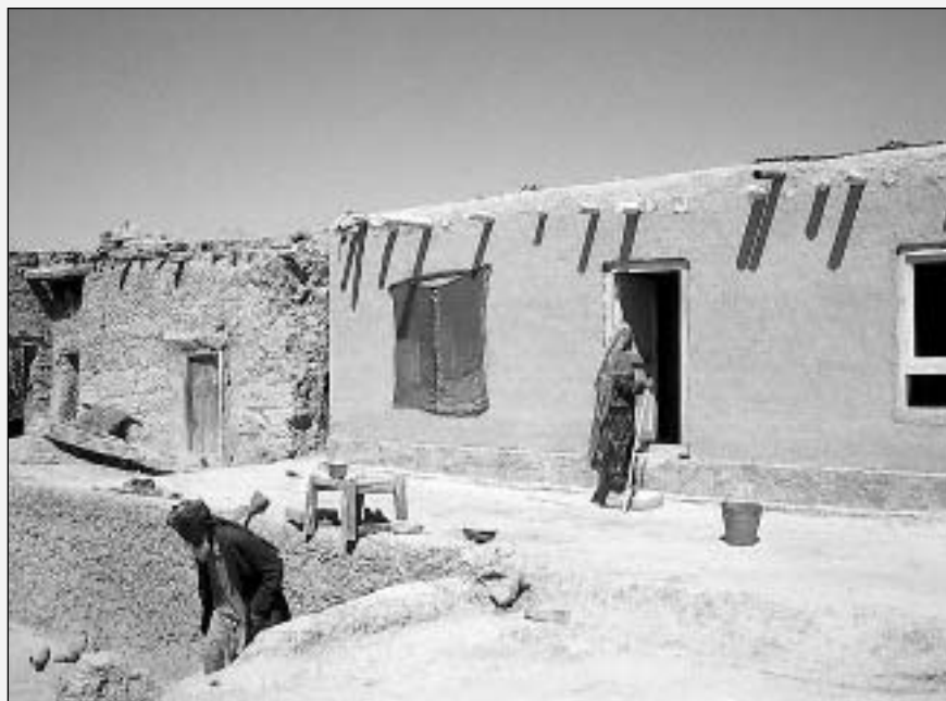
SFL's newly constructed temporary emergency shelter on the right, designed with earthquake mitigation measures, is a striking contrast to an existing shelter on the left in Baghlan Province (photo courtesy of SFL).
