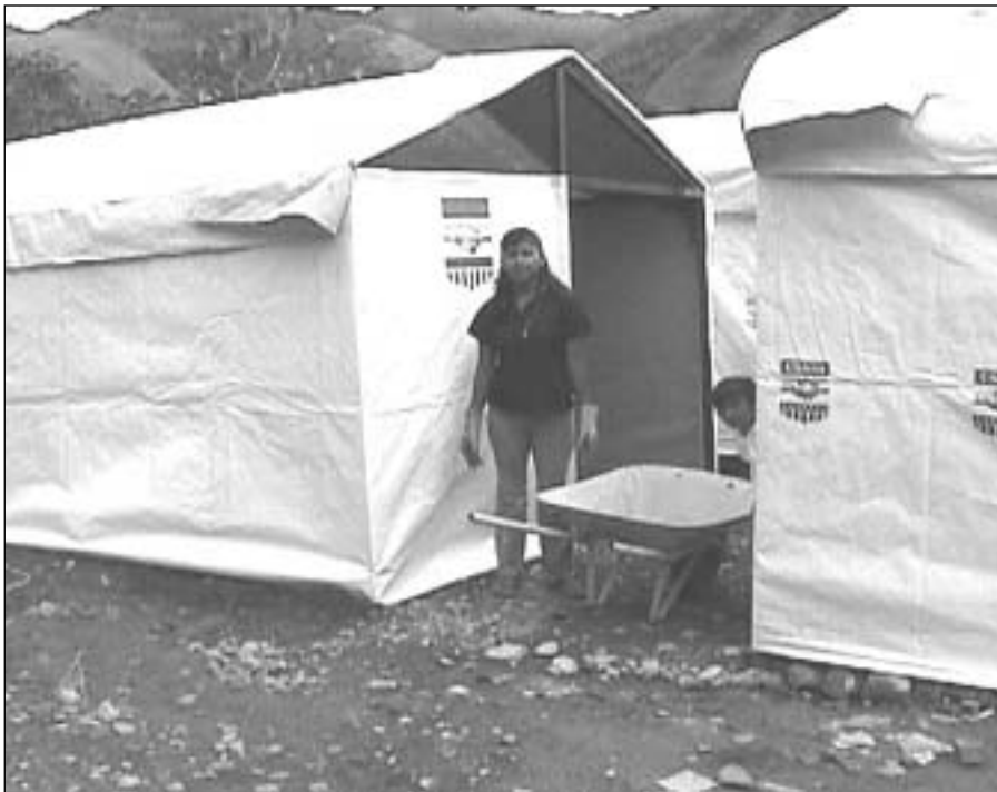
Temporary shelters were constructed in Chima, Bolivia, following a landslide that destroyed at least 150 homes (photo courtesy USAID/Bolivia).
