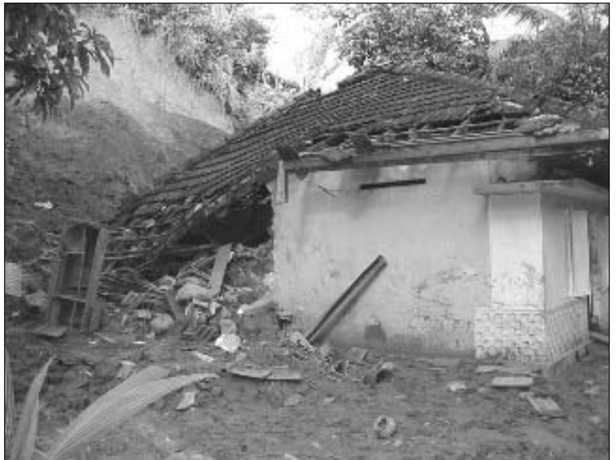
Landslides destroyed this house in Sri Lanka during the May flooding (photo courtesy of Chrisantha Jayakody, WVI).
