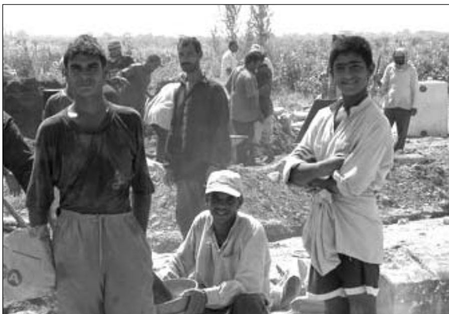
Local residents working on a school rebuilding project in Fallujah, Iraq (photo by USAID/OFDA).
