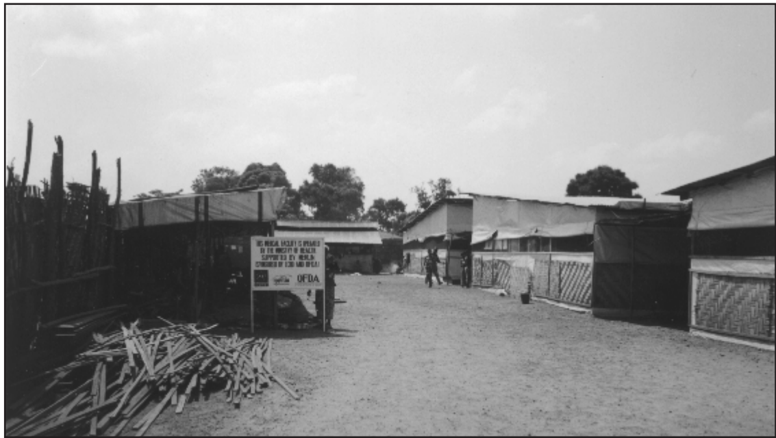
USAID/OFDA partially funded this emergency health care facility for IDPs in Kenema, Sierra Leone (photo by Sureka Khandagle, USAID/OFDA).
