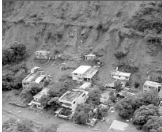
Hillside homes destroyed by landslides near Macuto in Vargas State, Venezuela (photo by Alejandro James, USAID/OFDA).
