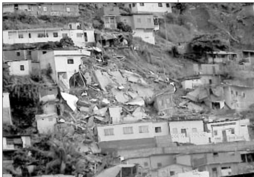
Hillside homes destroyed by landslides near Macuto in Vargas State, Venezuela. (photo by Alejandro James, USAID/OFDA).
