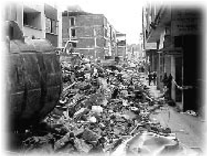
A street in Armenia, Colombia following the January earthquake (photo by Miami-Dade Fire and Rescue Team).
