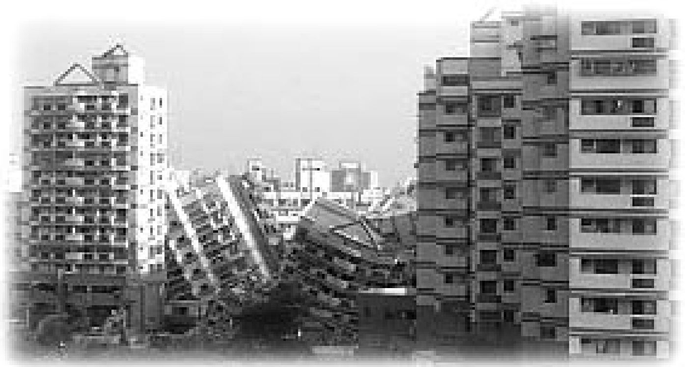
Two apartment buildings crumble to the ground in Toulun, Taiwan as a result of the September 21 earthquake (photo by Miami-Dade Fire and Rescue Team).
