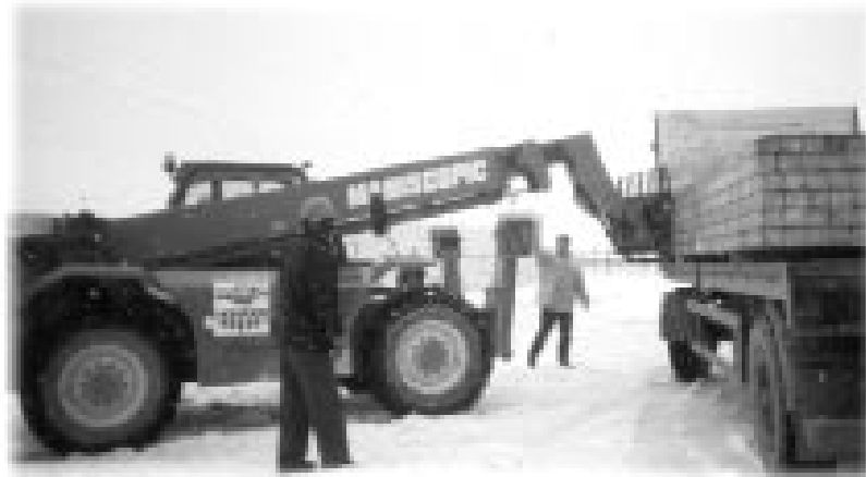
Lumber is off-loaded in the BHR/OFDA-funded emergency shelter materials depot in Gjilane (Ferizaj), Kosovo (photo by Jamy Bond, BHR/OFDA).
