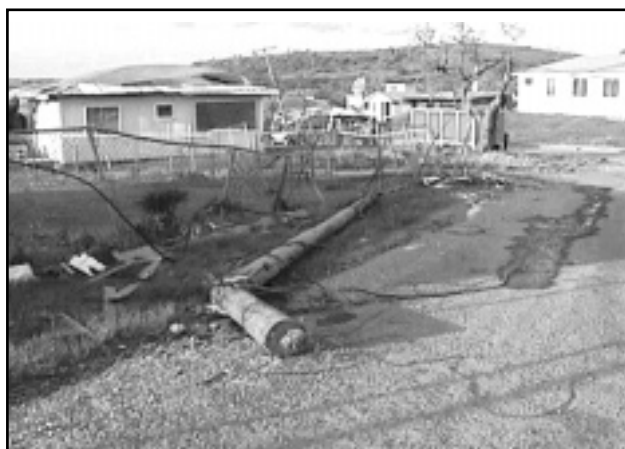
A downed utility pole in Antigua. About 50% of the telephone lines in Antigua sustained damage during the hurricane, and electricity was available only in the capital, St. John. (Photo by the Miami-Dade Fire and Rescue team)
