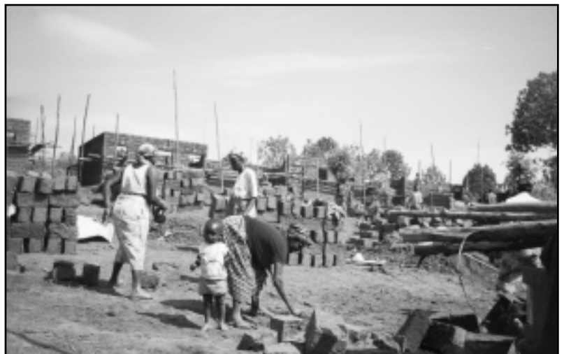
Women prepare earthen blocks for the construction of homes being built in Kimironko through a BHR/OFDA-funded shelter program. (Photo by Nina Minka, BHR/OFDA)
