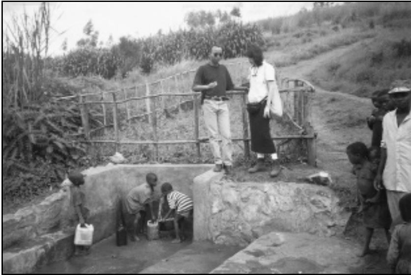
A protected spring built by IRC with BHR/OFDA-funding is inspected by BHR/OFDA's Regional Coordinator for the Great Lakes, Regina Davis-Tooley, and a local IRC representative. (Photo provided by Regina Davis-Tooley, BHR/OFDA)
