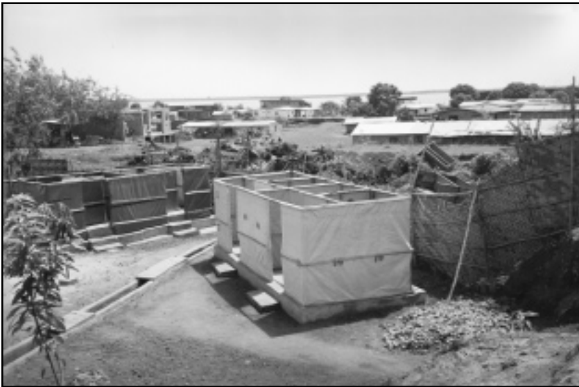
Latrines using BHR/OFDA-provided plastic sheeting are constructed in a village damaged during the conflict which ended in 1996. (Photo by Sureka Bacchus, BHR/OFDA)
