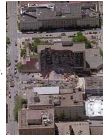
Alfred P. Murrah Federal Building, Oklahoma City After 5000 lb ANFO Truck Bomb
