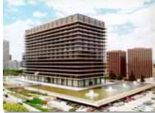
John Ferraro Building LADWP Headquarters Los Angeles, California
