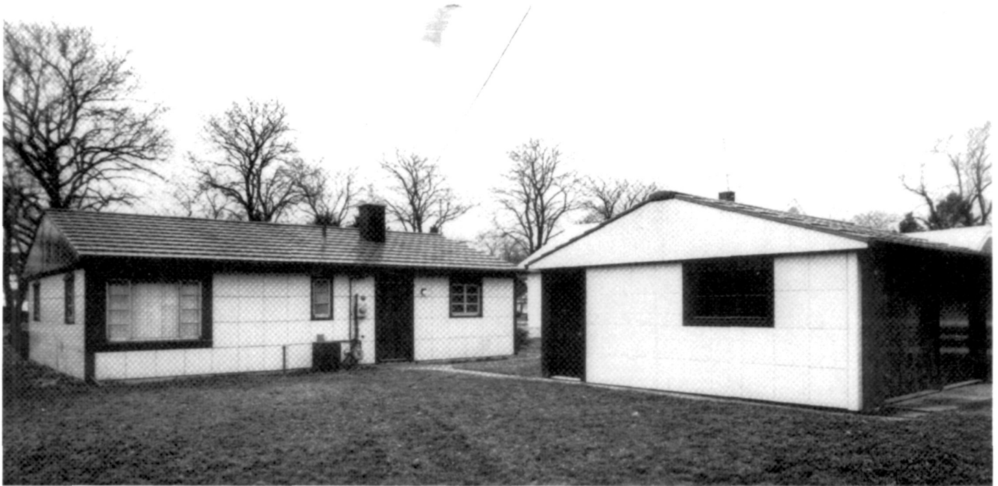
Completed in the spring of 1950, this pre-fabricated, all-metal Lustron House, Porter County, Indiana, was considered by many at the time to be the house of the future. (Beverly Overmeyer, April, 1992)
