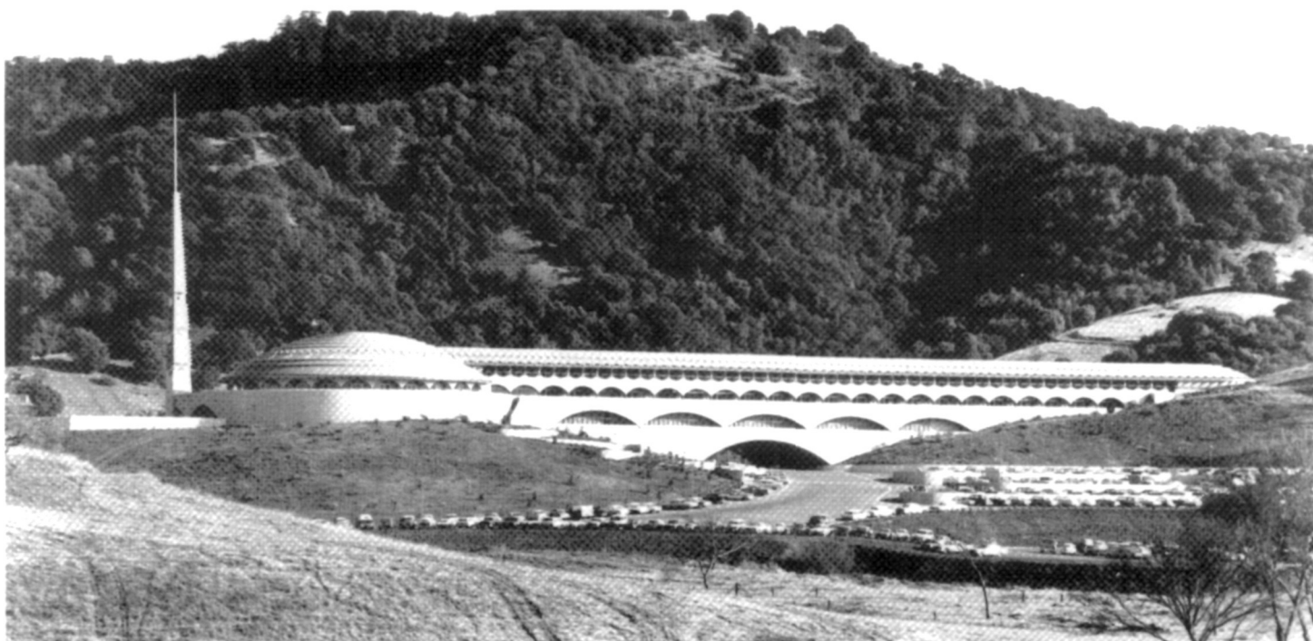
Frank Lloyd Wright's Marin County Civic Center, Marin County, California, completed in 1958, is an ideal government complex in a beautiful suburban setting. (Aaron Green, Woodbridge, 1990)
