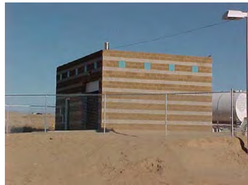
On-site Air stripper treatment building
