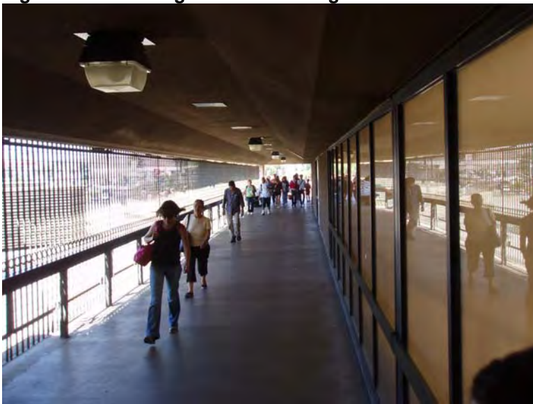
Figure 2-13: Existing Pedestrian Bridge
