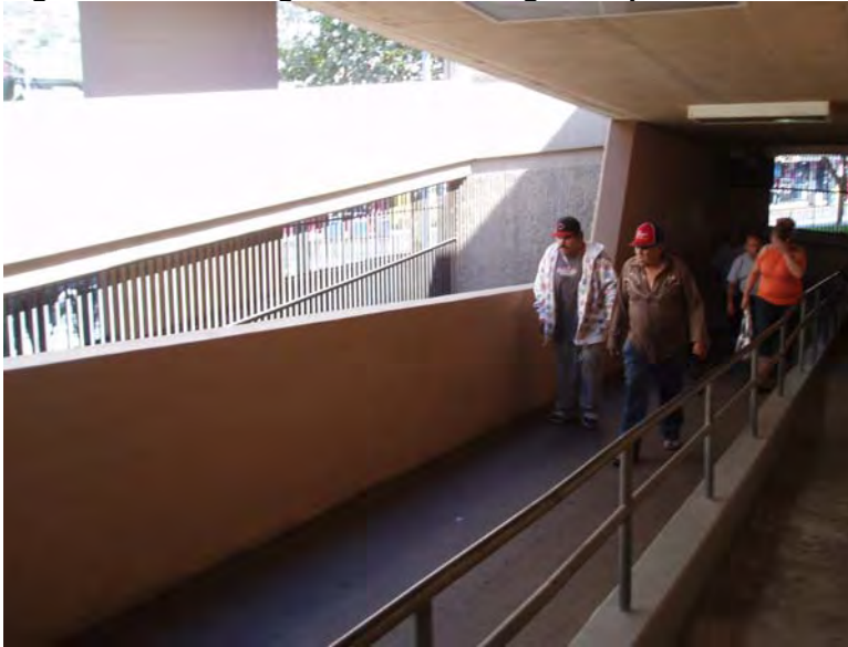
Figure 2-12: Existing Pedestrian Bridge Ramp
