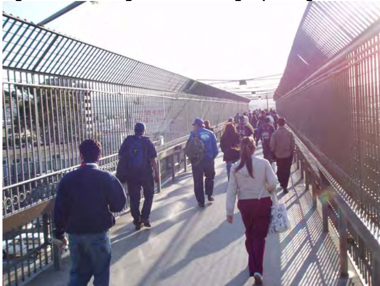
Figure 2-10: Existing Pedestrian Bridge Spanning Interstate 5
