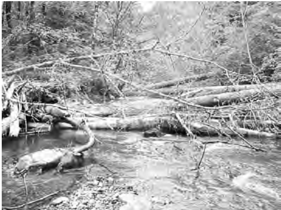
Figure 44. Alternative E would create stable in-stream structure on larger streams adjacent to mid-seral stands.
