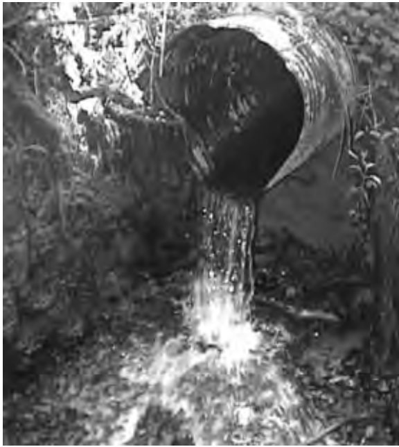
Figure 20. Under Alternative A, barrier culverts would continue to block access to potential fish habitat.
