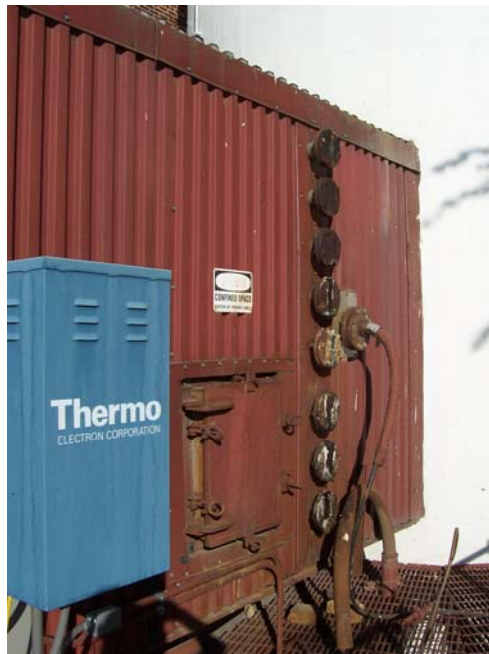
Figure 2-4. Test Port Locations for UI-10
