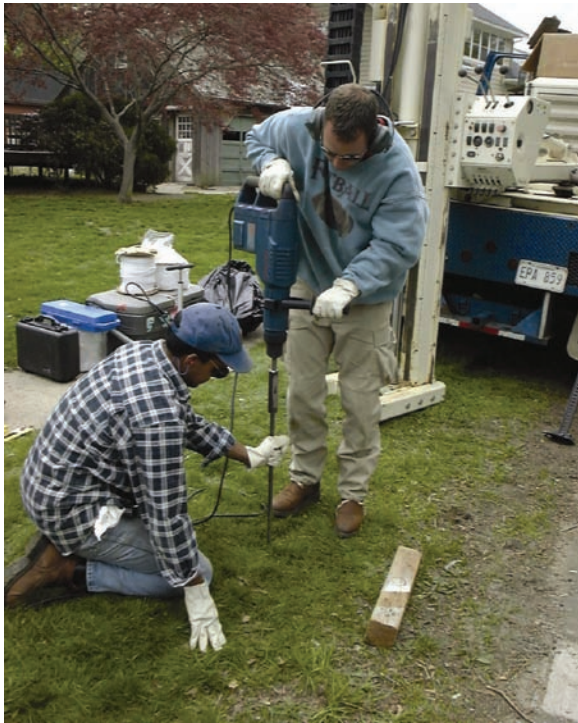
Figure 20. Photograph of hammering Retractable Tip and support pipe using a rotary hammer drill and the GVP extension drive adapter.
