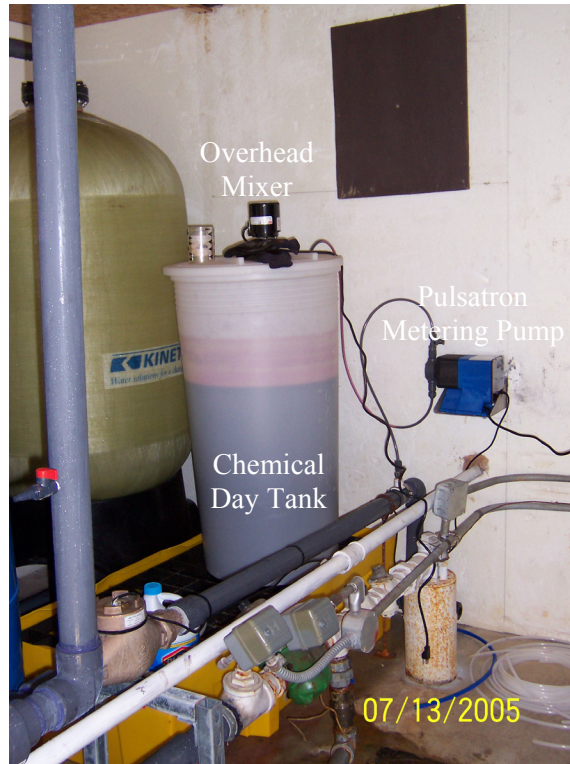
Figure 4-5. \text{KMnO}_4 Feed System
