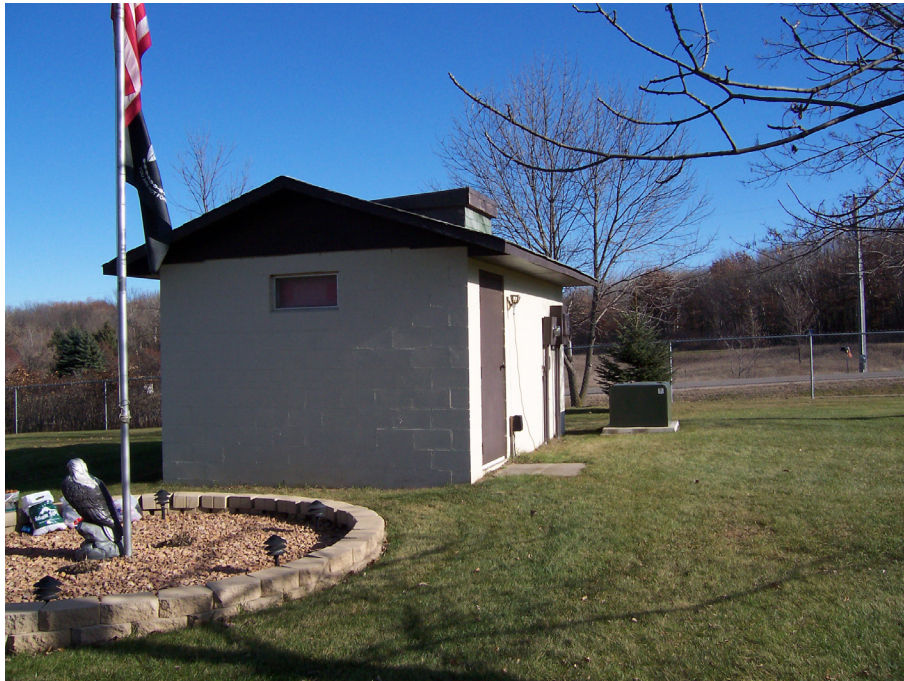
Figure 4-1. Preexisting Well House at BSLMHP, MN Site
