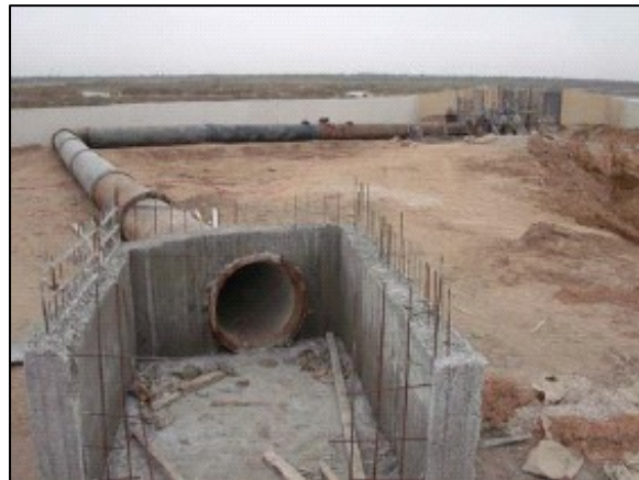
150,000 people will benefit from the sewage plant rehabilitation.
