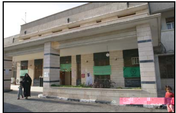
Renovated Health Clinic in the South Photo: Thomas Hartwell
