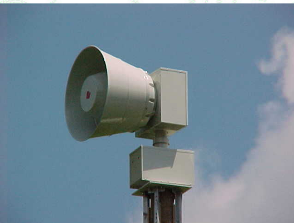
Above: A tornado siren. Sirens only alert people who are outdoors, and who are close enough to hear them.
