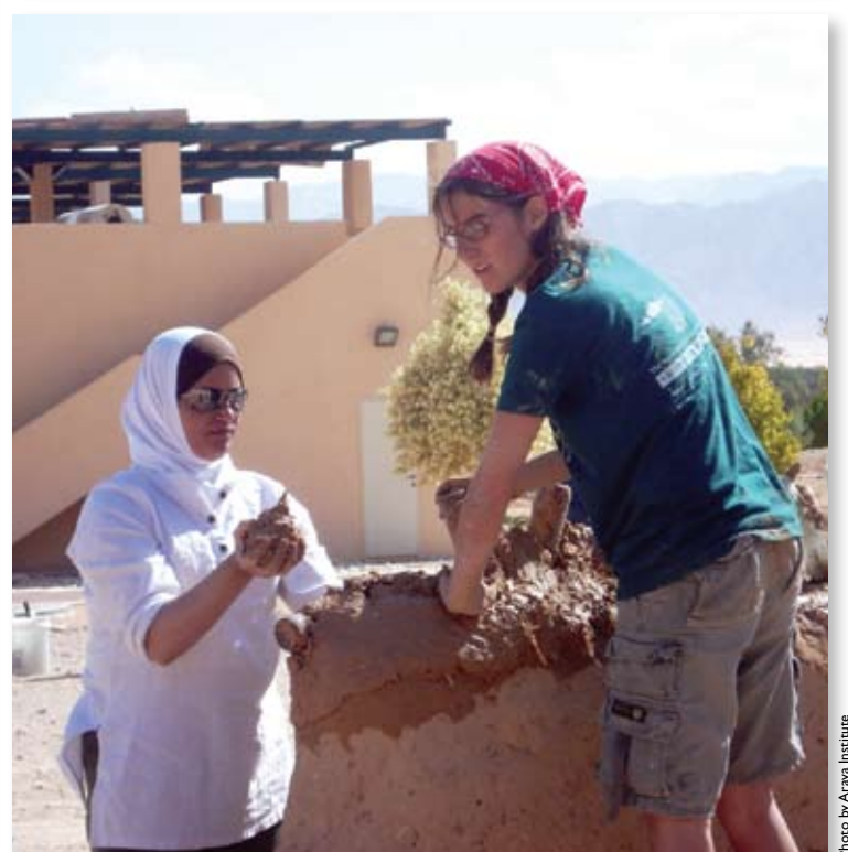
Students learn to make mud repairs on mud seats with Arava Institute dormitories in the background.
