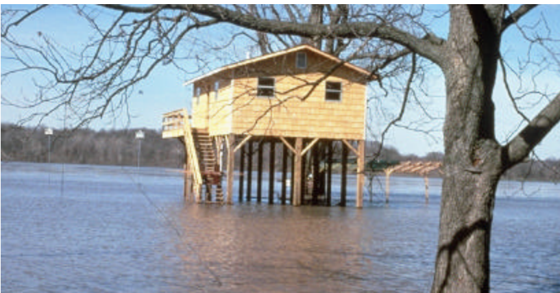
This house was elevated and the lower area was not enclosed. There was no flood damage to the structure.
