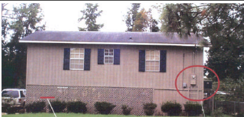
Flood protection elevation
