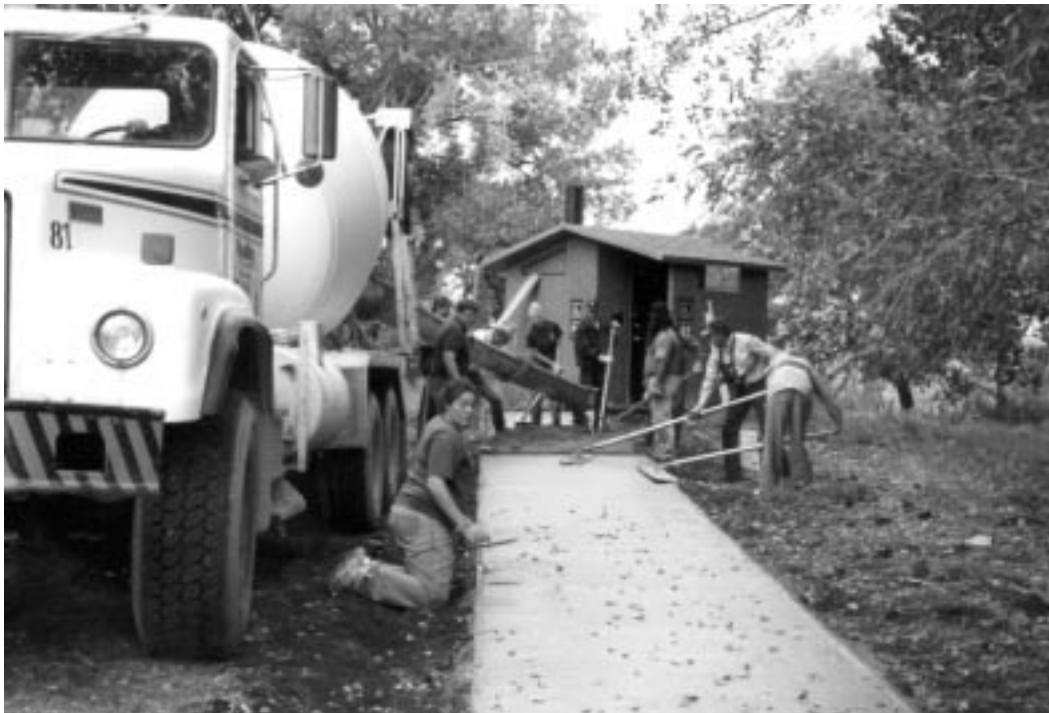
At Montana's Altman Confluence site near Billings, volunteers poured a 140-foot x 5-foot wheelchair-accessible sidewalk leading to a vault toilet; an extra 2-foot x 3-foot commemorative slab was also poured to allow National Public Lands Day volunteers to leave their signatures or initials. They indeed left their mark upon the land!
