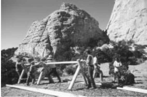
National Public Lands Day volunteers constructed a buck and pole fence to restrict OHV use in and around historic mining operation in Copper Globe Mine, Arizona.
