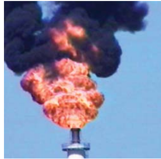
Flare at the Conoco Phillips Refinery in Rodeo
