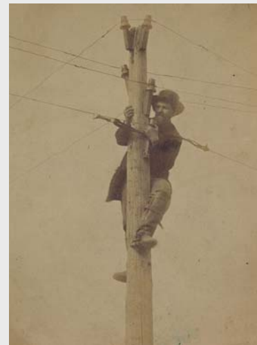
Lineman fixing a telegraph line, circa 1862. To reduce leakage of electrical current, telegraph line wires were tied to insulators attached to poles. Courtesy Library of Congress
