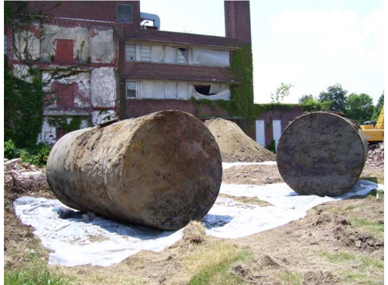
U.S. EPA's cleanup included excavation and proper disposal of underground storage tanks.
