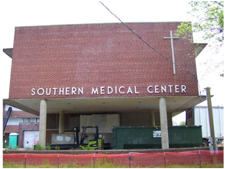
Cedar Street view of main entrance.
