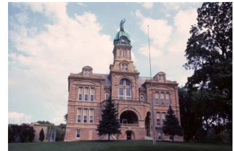
Blue Earth County Courthouse Mankato, MN
