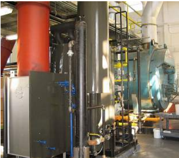
Ethicon Cornelia, GA Boiler Upgrade
