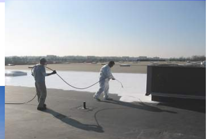
Healthcare Systems Memphis, TN Cool Roof Coating
