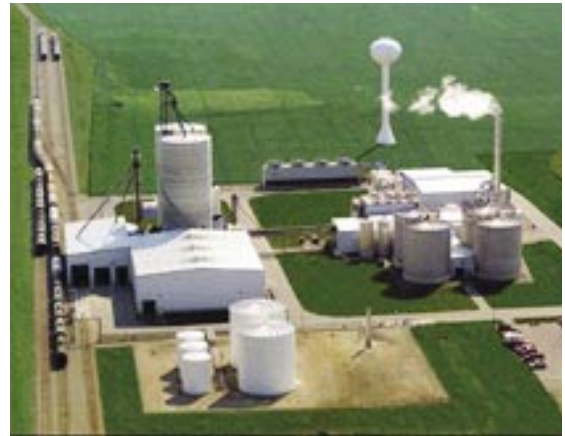
Midwest Grain Processors facility, served by Iowa Lakes Electric Cooperative, expanded from a 5-MW load to a 9-MW load. (Photo by ILEC)
