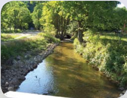
The restored creek runs through the proper channel. The boards, blocks and concrete dam were removed.
