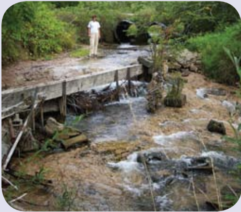
Dair Creek was re-routed and forked in the late 1800s to support Dair Mill. A dam was also built, impeding stream flow and fish passage.
