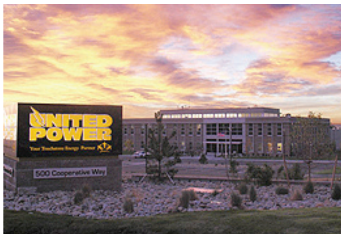
United Power's headquarters in Brighton, Colo., enjoys year-round comfort and energy savings because it is heated and cooled with 35 all-electric geothermal heat pumps. (Photo by United Power)
