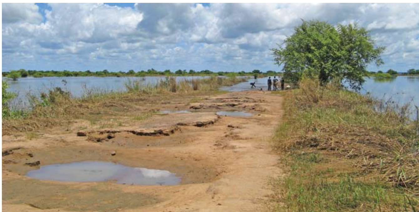
A road damaged by flooding impedes travel in Mopeia, Mozambique (Photo by Tresja Denysenko, USAID).
