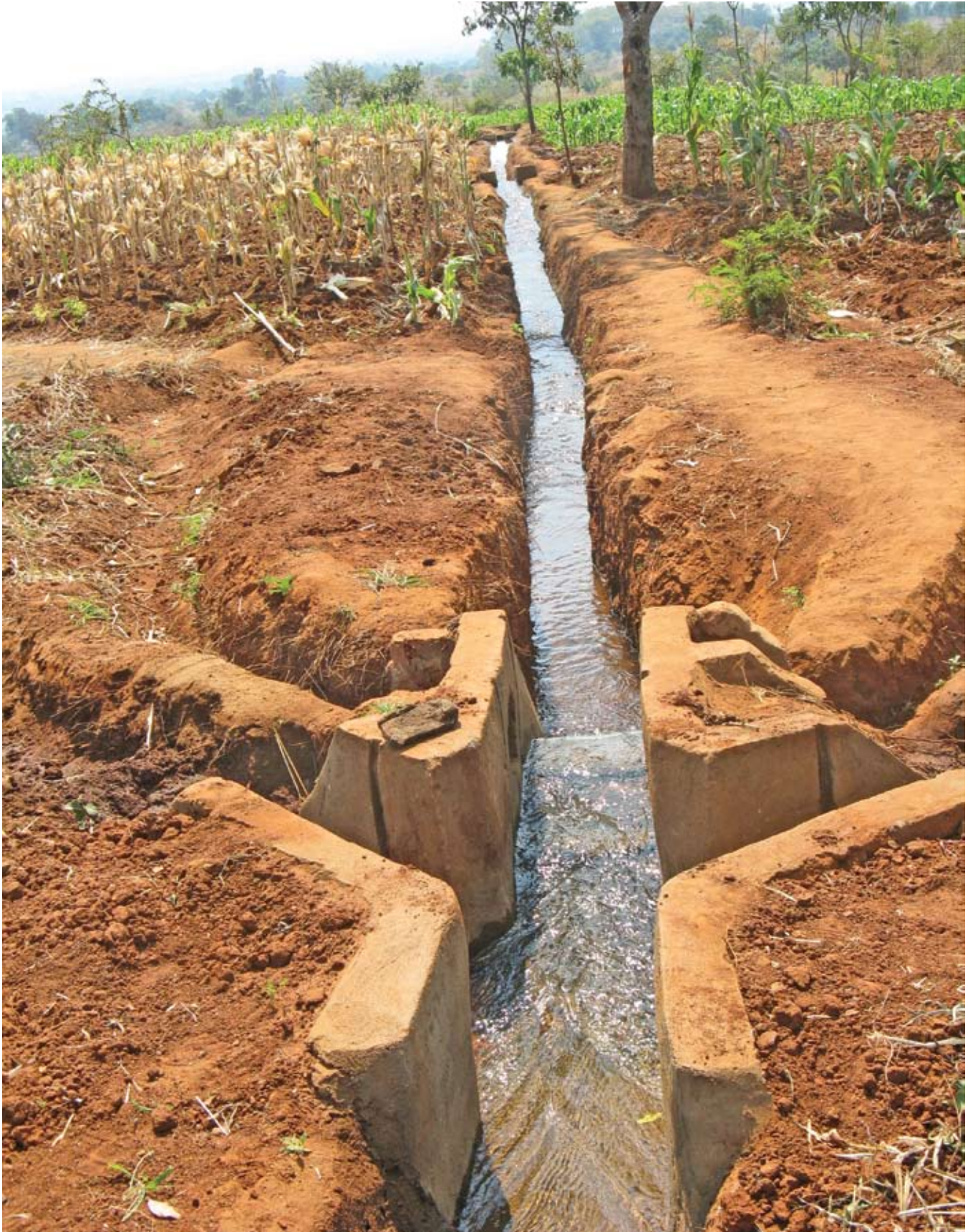
Constructed with OFDA support, a canal channels water to nearby crops in Malawi (Photo by Alexandra Riboul, USAID).
