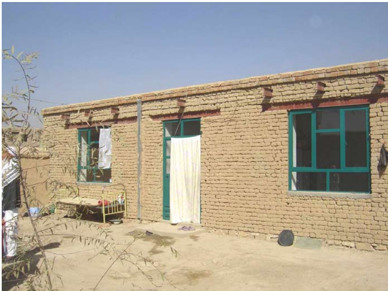
A seismic-resistant shelter reduces the impact of earthquakes on residents in Afghanistan (Photo by Charles Setchell, USAID).
