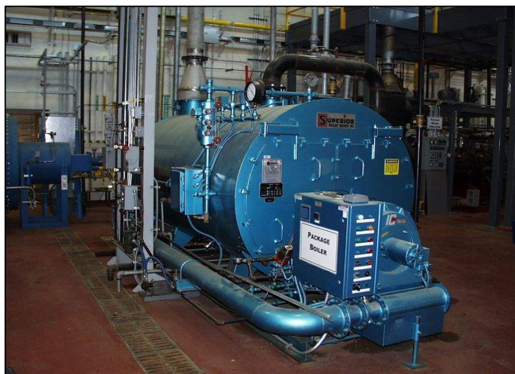
Figure 3-1. Wetback Scotch Marine Package Boiler
