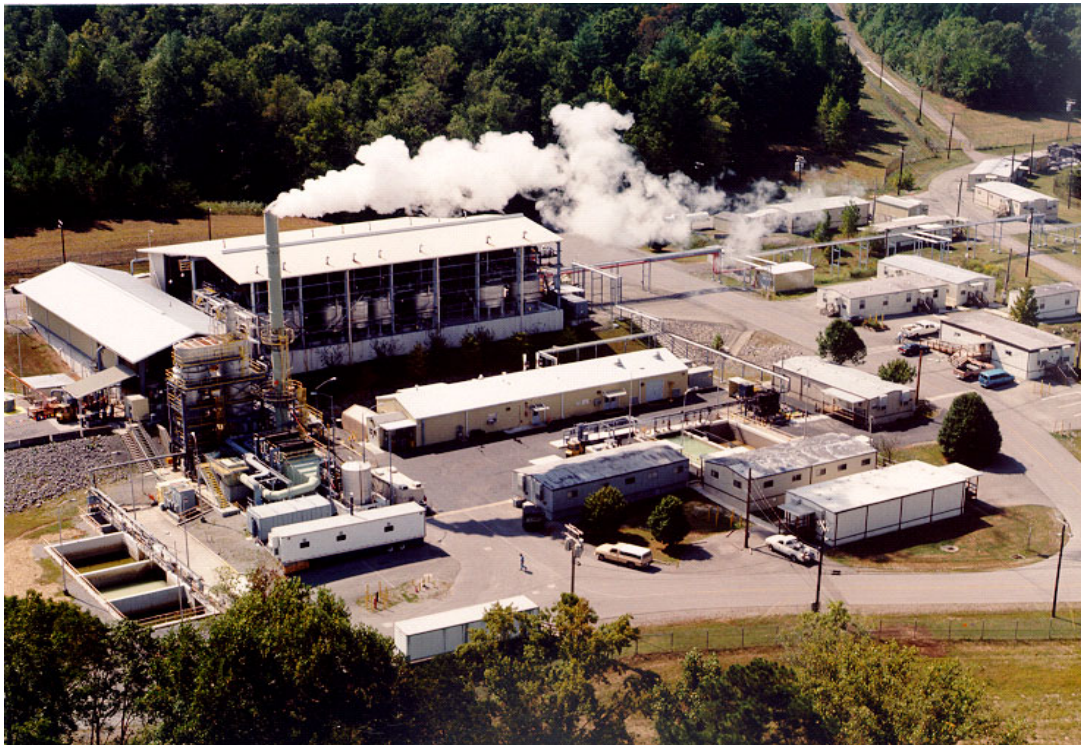
Figure 3-2. Overview of TSCAI Test Location. The incinerator stack is at left, with waste feed area behind the stack. The trailers housing the mercury CEMs for this test were located in the foreground at the base of the stack.
