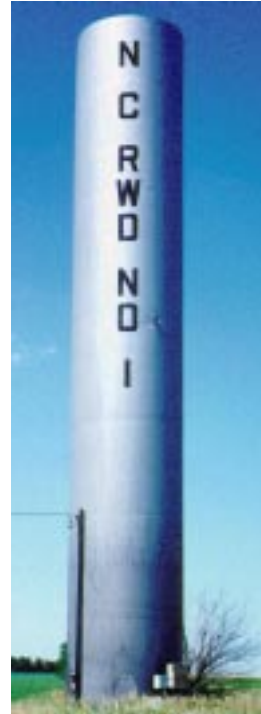
Figure 4.16 Rural Water District standpipe (Nemaha County).
