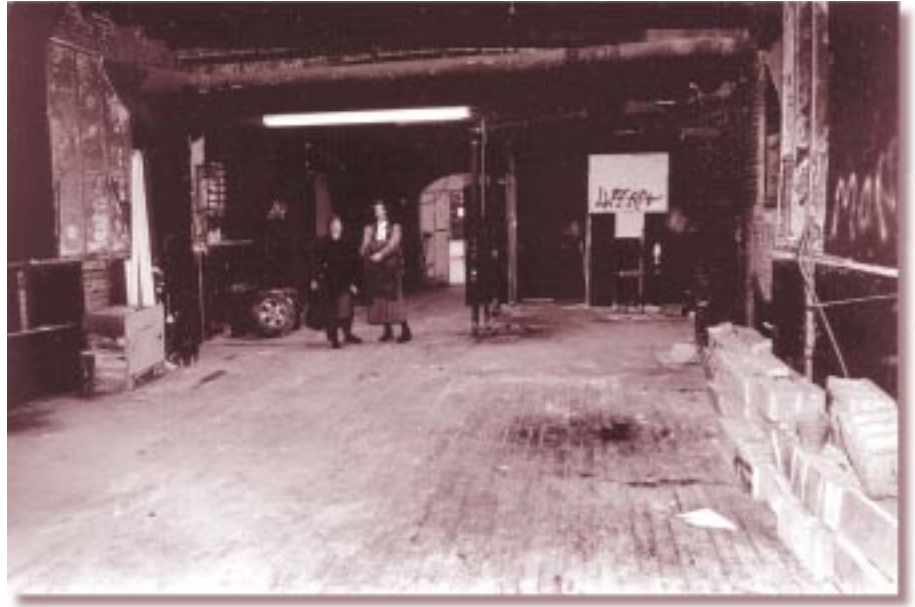
Site of La Bodega de la Familia before its renovation.
