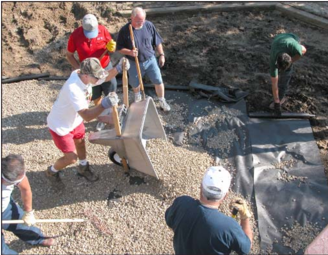
Figure 3—Placement of drainage fabric and rock on playground subsurface.
