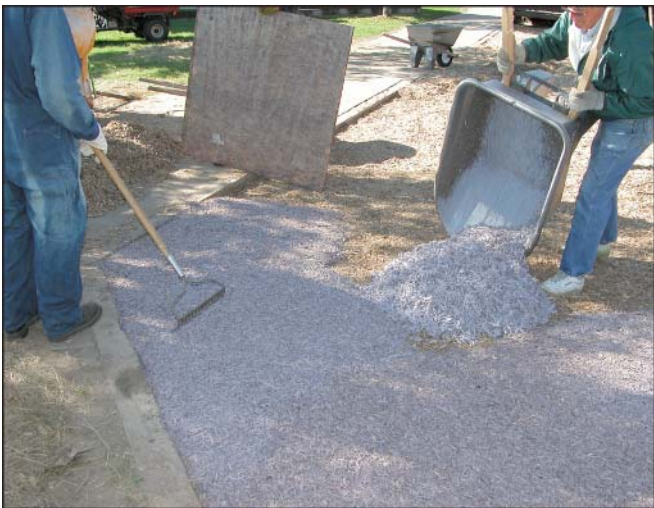
Figure 7—Leveling and compaction of binder–EWF mixture.
