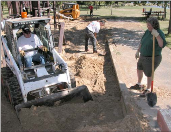
Figure 2—Removal of sand from existing playground surface.
