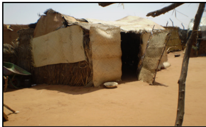
3.1b: Typical house construction in Otash Camp
