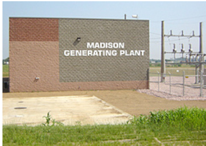
The city of Madison built this 10-MW powerplant as part of an agreement with Basin Electric Power Cooperative. The facility provides stand-by generation for the municipality and emergency power to Basin. (Photo by Madison Electric Utility)
