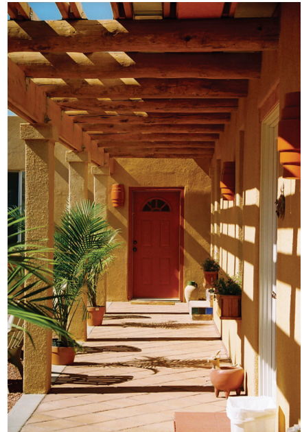
Navajo architecture students built the first house using Navajo Flexcrete blocks. Traditional features like this courtyard act with the block's insulating properties to keep out the desert heat. (Photo by Navajo Housing Authority)
