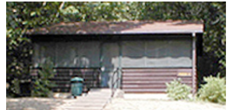
NPPD is providing partial funding through a grant to Ponca State Park, Neb., to build a guest cabin like this one with energy-efficient construction, lighting, heating and cooling controls and complete on-site waste disposal and treatment. (Photo by Nebraska Game and Parks Commission)
