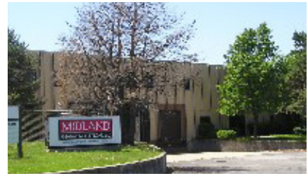
BPU helped Midland Pharmaceutical reestablish electrical service and update of a former pharmaceutical facility. (Photo by Midland Pharmaceutical)
