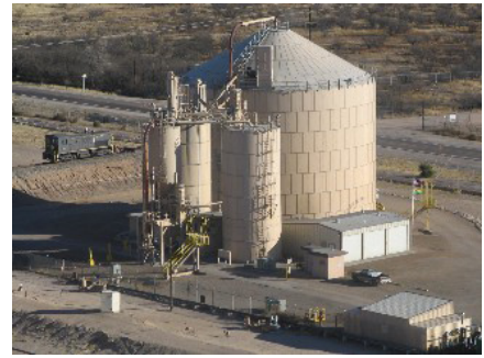
The Apache Station coal-fired powerplant produces thousands of tons of fly ash annually that AEPCO markets to concrete manufacturers. (Photo by Boral Material Technologies)
