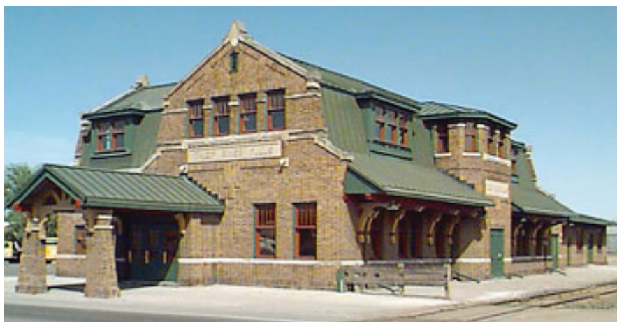
The Thief River Falls City Hall is one of three city facilities to install a geothermal heat pump. (Photo courtesy of TRF Utilities)
