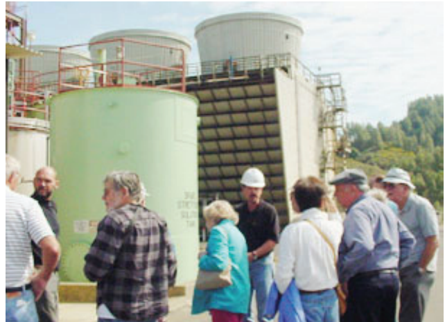
Geothermal Facilities Manager Murray Grande (center in hard hat) of Northern California Power Agency leads Alameda P&T customers on tour of NCPA's geothermal plant No. 1 located in Middletown, Calif. (Photo courtesy of Alameda Power and Telecom)
