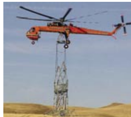
A helicopter lifts a bridge section into place during the construction of the Path 15 Upgrade. The project is on schedule for completion in late 2004. (Photo by Dave Christy.)
