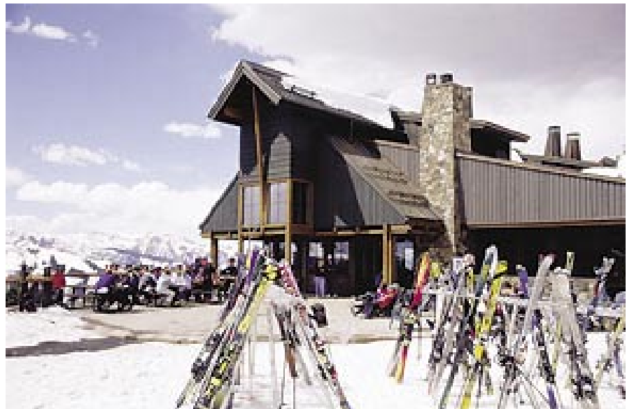
The Sundeck restaurant at Aspen ski resort was one of the first green building projects in the world to receive LEED certification. Aspen Ski Company hopes its recently completed Snowmass Golf Club will earn a gold certification. (Photo courtesy of Hal Williams)
