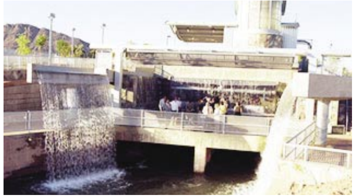
Arizona Falls, a low-impact hydroelectric facility built on the Arizona Canal Network, contributes to Salt River Project's renewable portfolio, and demonstrates renewable energy in action. (Photo courtesy of SRP)
