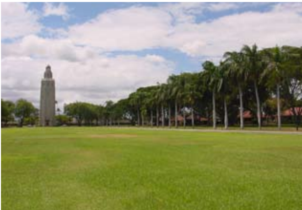
Hickam Historic District's central grass mall with the Hickam Water Tower, known as "Freedom Tower" (Photo courtesy U.S. Air Force)
