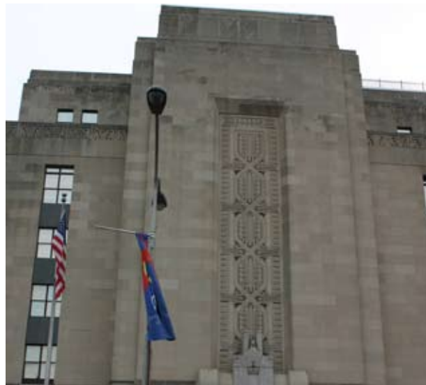
The Main Post Office in Philadelphia is listed on the National Register of Historic Places. It will be redeveloped using historic preservation tax incentives.
