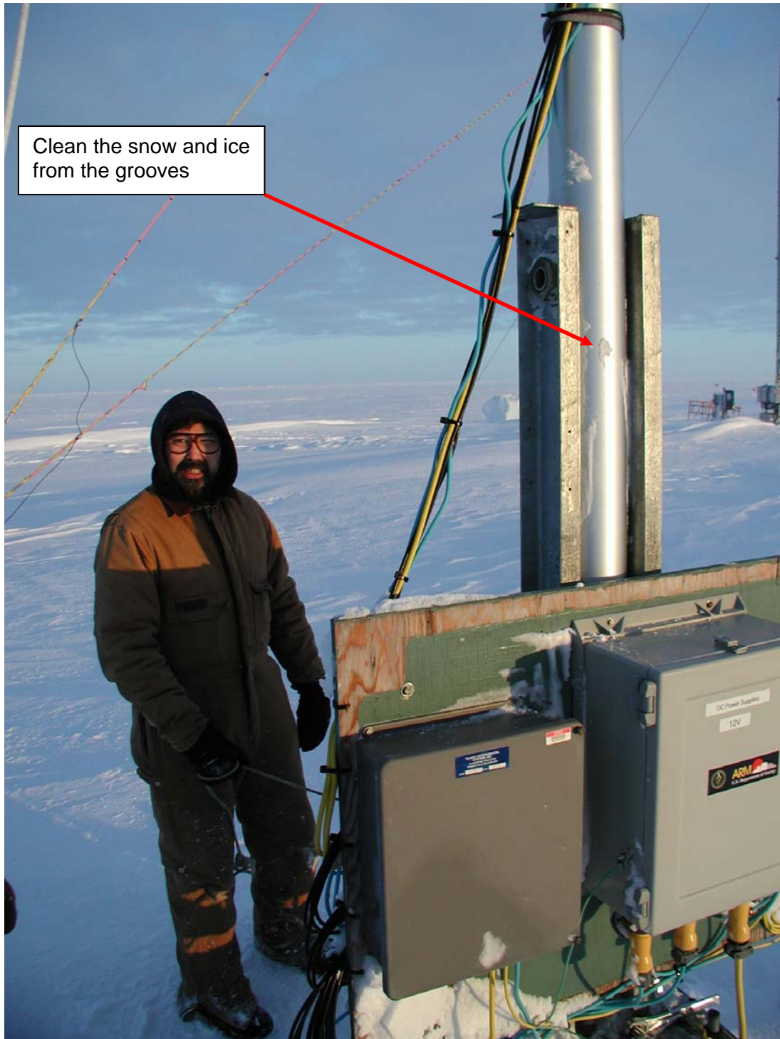
Figure 1 The hinge section of the tower.
