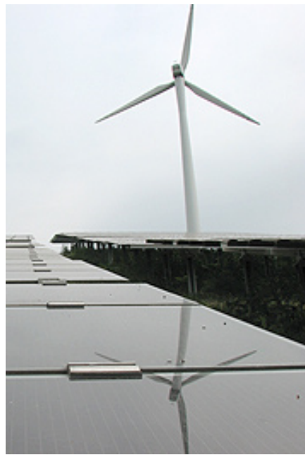
The SEPA delegation visited a landfill powerplant site in Germany where this solar array and wind turbine are co-located. (Photo by Mike Taylor, Solar Electric Power Association)
